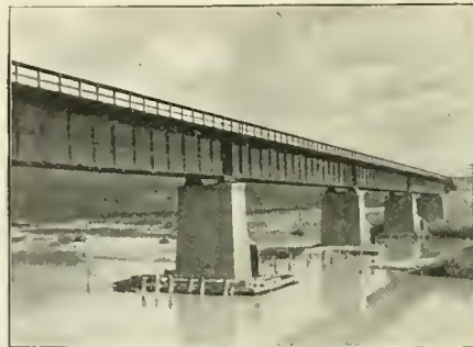
U. P. NEW BRIDGE AT FORT STEELE, WYO.
